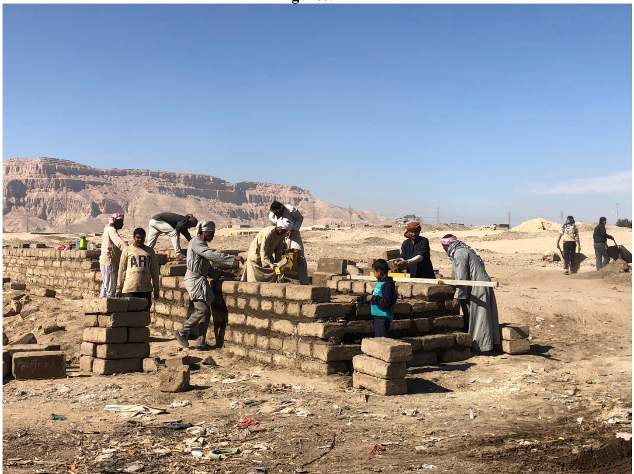
Fig. 1 Restoration work on the North Palace and Enclosure Wall, to preserve the archaeological remains and act as a protective barrier to the site (Photograph Nicholas Brown)
